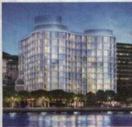
The curvaceous 160 Leroy will rise along the West Side Highway.
